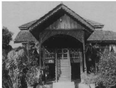
The Malay vernacular houses are raised on timber stilts and made of local materials such as timber, bamboo, rattan and leaves. They usually have pitched roofs, verandahs in front, high ceilings and many big openings for ventilation purposes. Their shapes and sizes are different from state to state.
