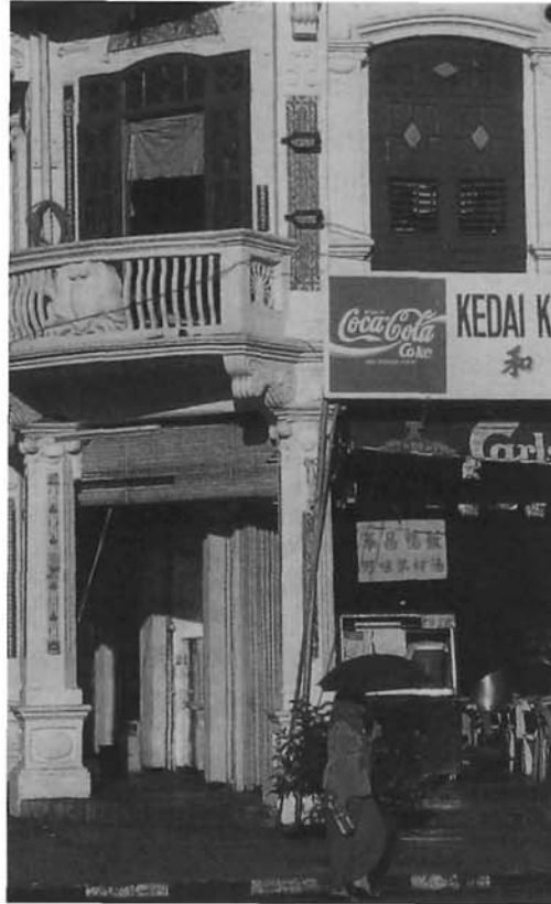
The Southern Chinese terrace houses and shophouses are the two most common buildings found in many urban areas in Malaysia. Each building is connected to several other houses to form a block with a street-level porch in the front. Building materials such as brick, plaster, concrete and timber are commonly found in the buildings.
